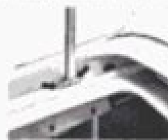
Fig. 5.1d: Straps that hold the roof cable in place
