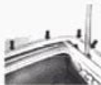
Fig. 5.1b: Strip that holds the bottom of the roof panel in place
