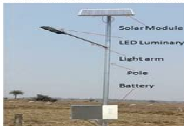
Figure 1 Stand alone Solar streetlight
